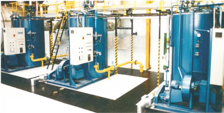
3 x Model 2500 RR VPX Babcock Wanson Steam Generators
