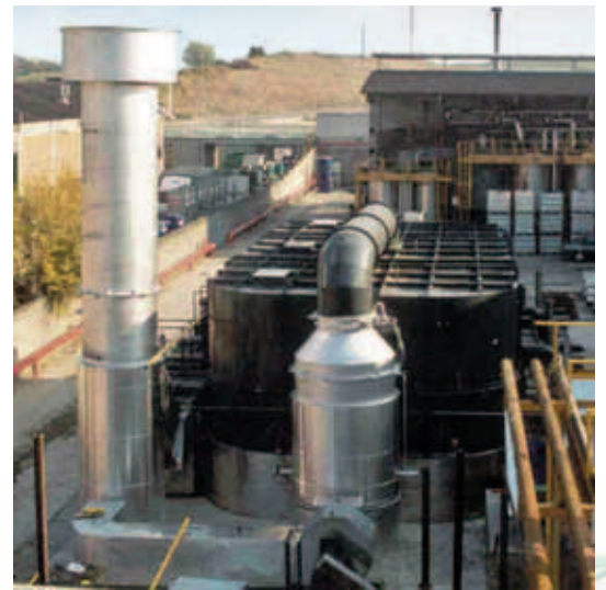
Fabric coating • 50,000 Nm 3 /h Thermal fluid heat recovery
