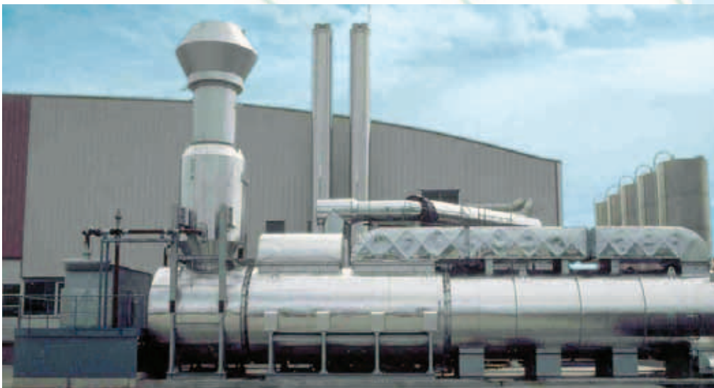
Aluminium foil printing. Effluent gas • 45.000 Nm 3 /h Thermal fluid heat recovery.
